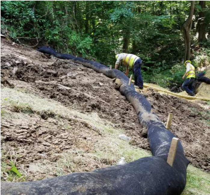
Silt socks placed on a hillside to prevent erosion downstream. Source: "Erosion Control." Fossil Rock Services, October 25, 2019. https://fossilrockservices.com/erosion-control/ .
